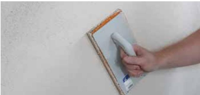
**5** After sufficient setting, the plaster is floated with a wooden or plastic float and can be finished over with a sponge float.
