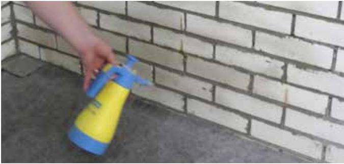
**1** After deep cracks and surface irregularities have been leveled out with KÖSTER Repair Mortar, the area is primed with KÖSTER Polysil TG 500.
