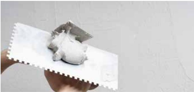
**3** KÖSTER Thermal Restoration Plaster is mixed into a workable mortar, and the first layer is thrown on and struck smooth.
