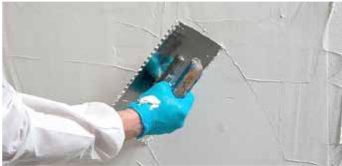
**4** KÖSTER Glass Fiber Mesh is embedded in the surface of the first layer, and the second layer of KÖSTER Thermal Restoration Plaster is applied.
