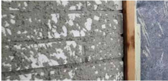
**2** KÖSTER Restoration Plaster Key is applied in a layer thickness of max. 5 mm with a coverage of approximately 50%.
