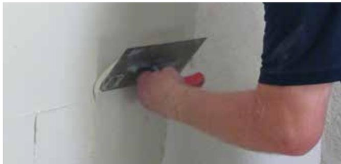
**6** KÖSTER Hydrosilicate Adhesive SK can be applied in a layer thickness of up to 2 mm to smooth the surface for a very smooth appearance.
