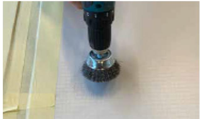
After preparing the crack and priming it, apply the first layer of KÖSTER MS-Flexfolie on top the primer, then adhere the KÖSTER Superfleece 10 cm wide, centered over the crack while it is still fresh. Slightly press it and fully cover it with a second coat of the KÖSTER MS-Flexfolie. Allow 6 to 8 hours to cure before starting the application of the area waterproofing.
